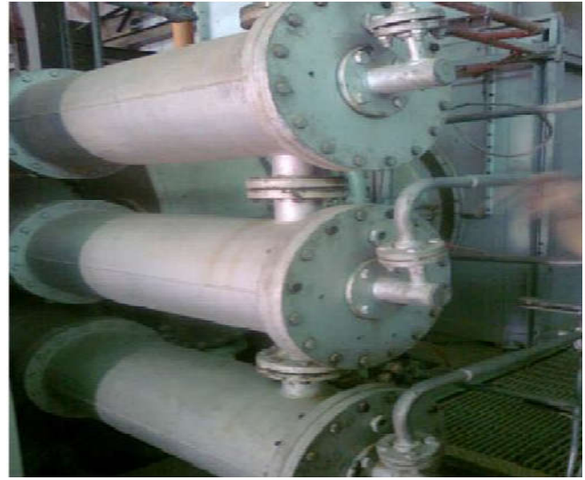
Figure III.4 : Chamber de combustion de la turbine TG GE 50001P
