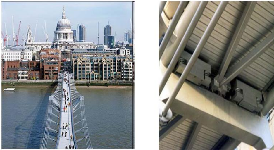
Figure 1.17 : Vertical TMDs installed under the deck of the Millennium footbridge in London
