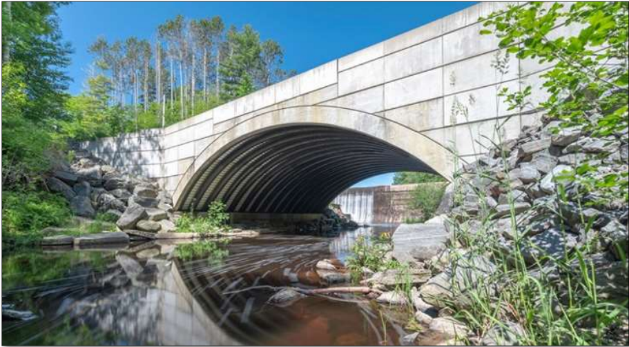
Fig 2. 3: AIT Bridges uses a braided fiber-reinforced polymer (FRP) tube filled with concrete
