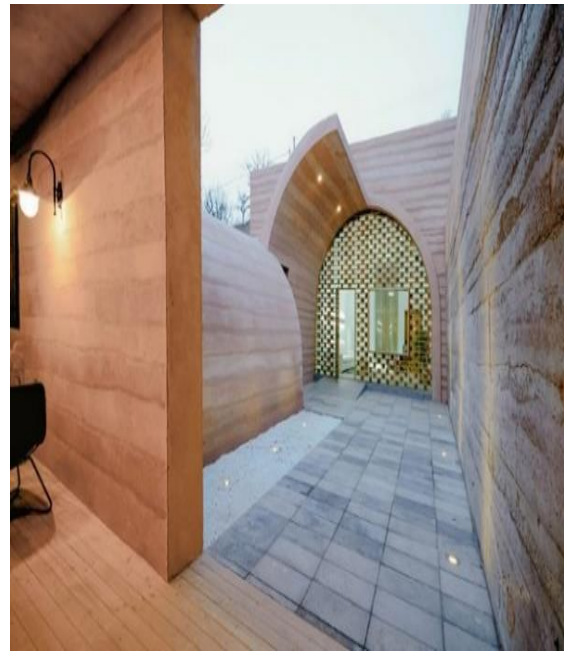
Figure I.3: Contemporary house made of rammed earth, China.
