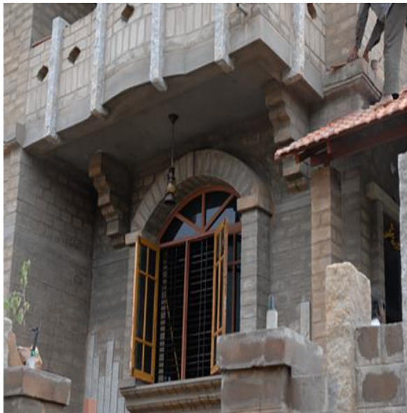
Figure I.4: Building with compressed earth blocks (CEB), India [19].
