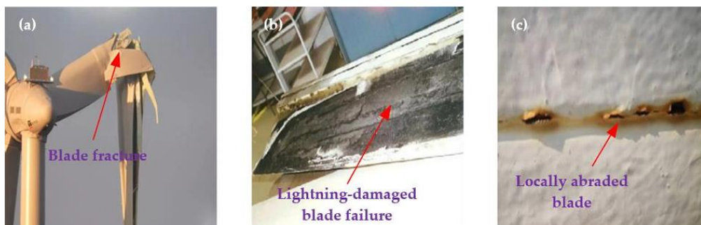
Figure 8: Common blade failure modes.[14]
