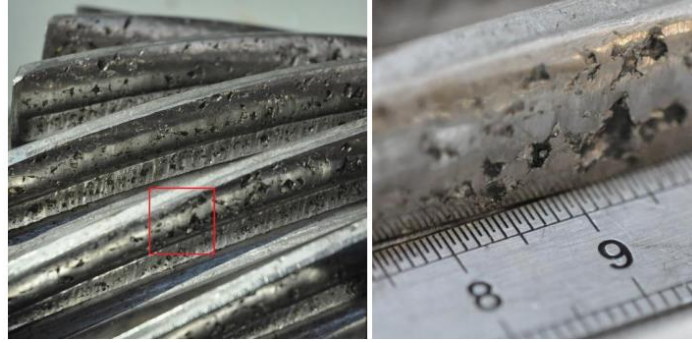
Fig. II. 2: Observation of pitting that spreads and causes flaking.
